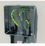
The earth from the mat can then be connected to the earth from the incoming supply by using the earth terminal in the back box. If using a plastic box with no terminal then a terminal block can be used.
