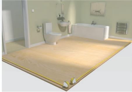
First measure the area to be heated in sqm (do not include the area taken up by fixed objects such as baths/showers and kitchen units), then divide this area by the length of the cable shown on the drum. The cable is 170 watts per linear metre so a 1350 watt kit contains 79 metres of heating cable. The spacing is calculated by dividing the total sqm of the area to be heated by the cable length in metres (see example below).
