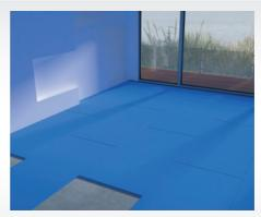
(**DO NOT** use XPS insulation boards on wooden sub-floors) (**DO NOT** use EPS insulation boards with this heating system)
